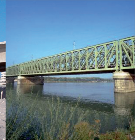
Railway Bridge Tulln, Austria
