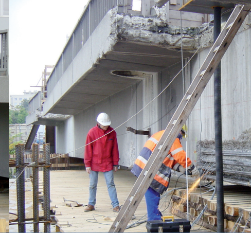
Uncovering of prestressing
