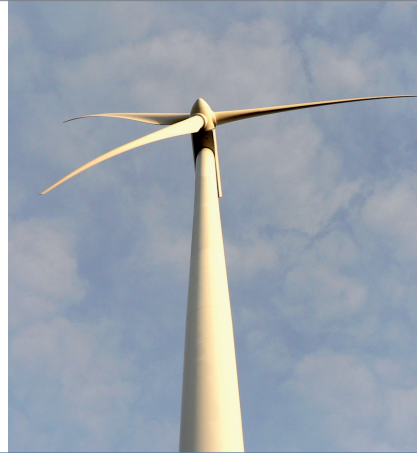
Wind power plant, Germany
